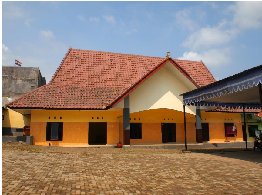
Gambar 3.1-4. Gedung SMA Bahrul Maghfiroh
