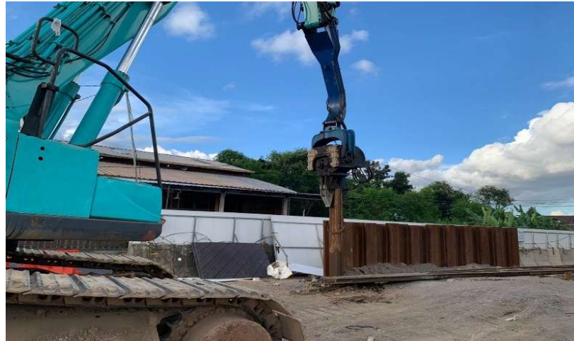
Gambar 4. 4 Proses Pancang Steel Sheet Pile
